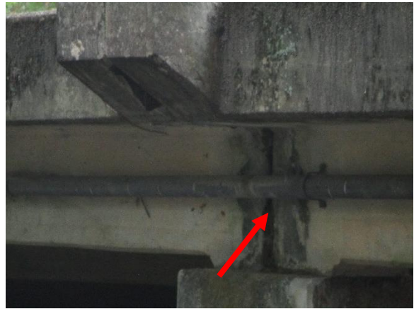
Photo 4. Expansion Joint Board
